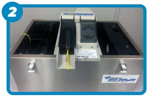
Unlatch and remove Inlet/Outlet covers and Electrical Assembly from Big Dipper Tank
