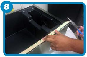
With residue removed, lay new gasket on front edge of unit and cut to length. Do NOT stretch
